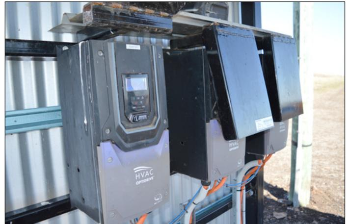
*Subtle adjustments to the variable frequency drives (VFDs) that operate three electric pump motors on Adam McVeigh’s Macalister farm have saved power input and costs.*
