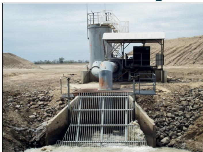
Figure 1: Large mixed flow pump used to lift floodwater and tailwater into irrigation channel (left background) and large earthen storage (right background).
